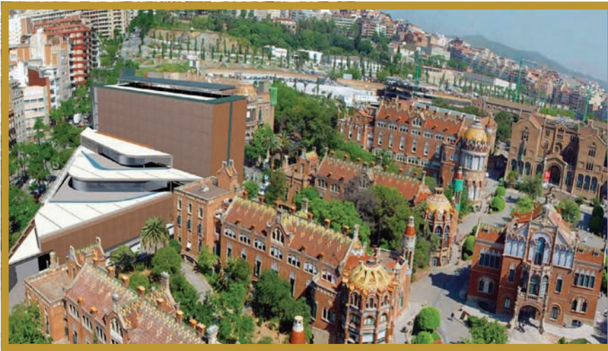
Fundació Puigvert is expanding its premises to build more clinical laboratories.
